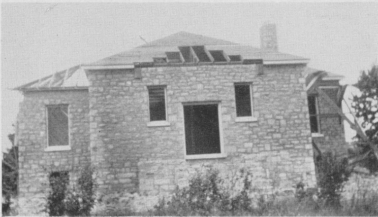
ON THE WAY TO COMPLETION
